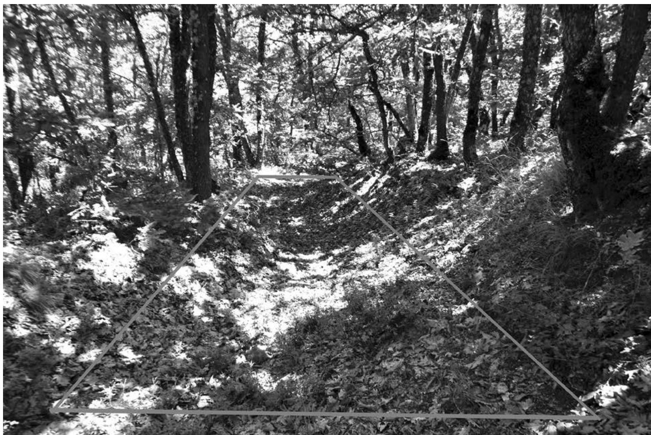
Figure 16.17. Guerrilla Hospital near Kottas village. Traces of the undercut chambers in the dense vegetation. The line indicates the original plan of the construction (photo by authors, 2019).
